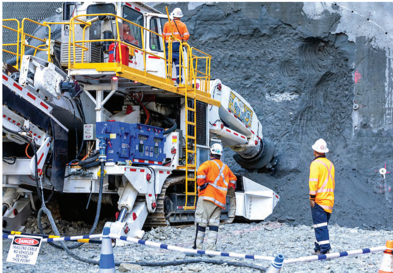
The roadheader at work.
